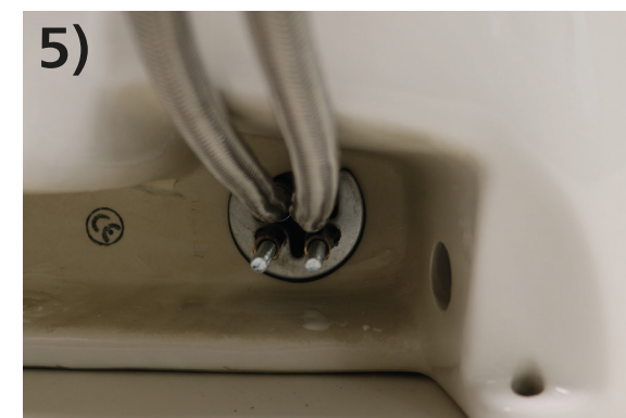
5) Position rubber washer over flexitales and bolts, followed by the metal washer. Use bolts to secure tap in place.
